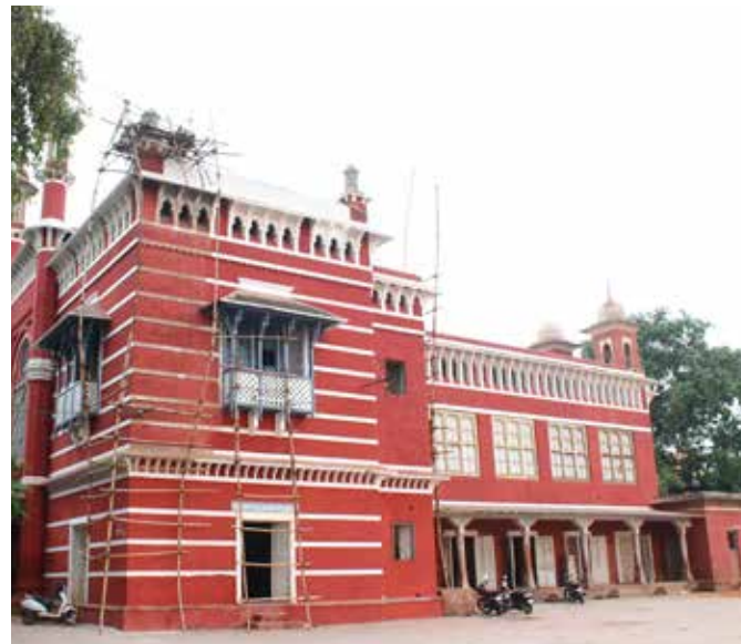
Cleaning and paintwork of the facade of Town Hall- 2016
