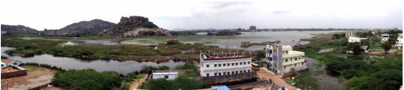
Bhadrakali lake- Before Foreshore Bund
