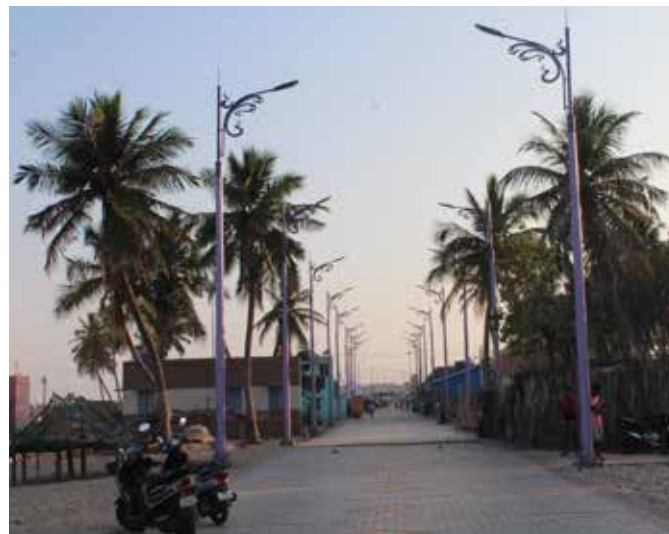
Erection of Heritage Street Lighting at Saparapathai street
