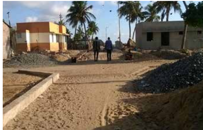
Saparapathai street- Before erection
