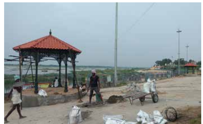
Street furniture under installation
