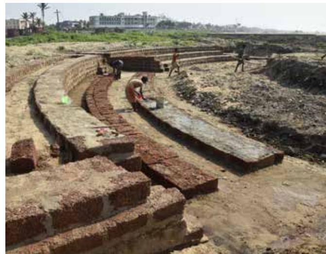
Development of landscape garden by using treated water from waste water treatment plant at Bankimuhan, Puri
