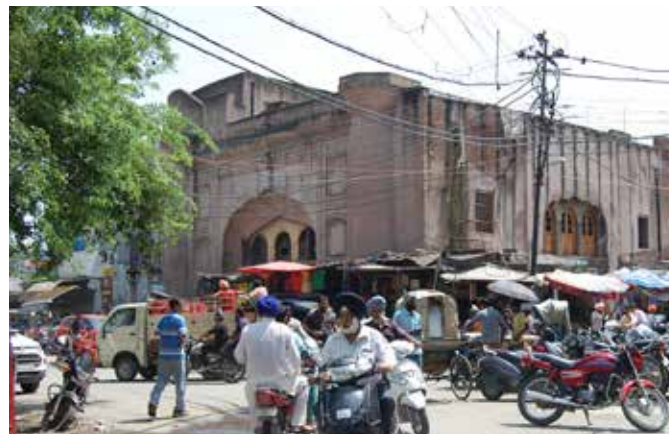
Current activity around the historic gate
