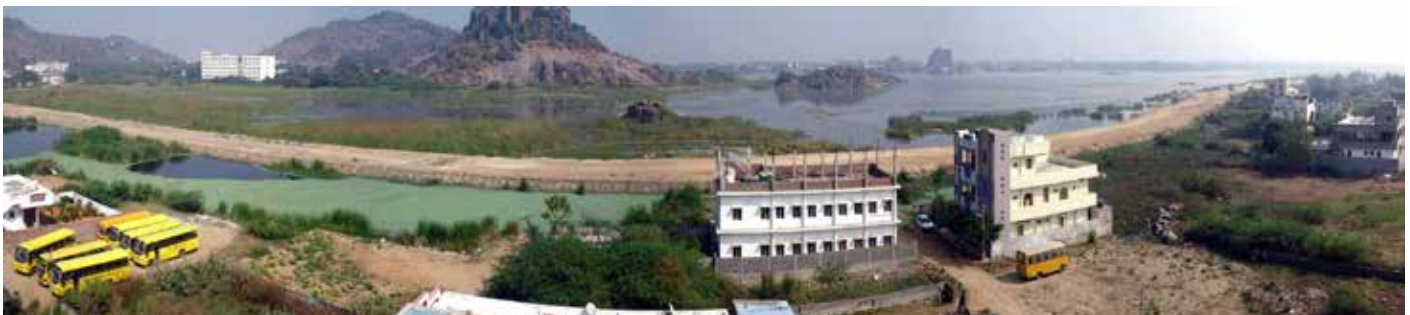
Bhadrakali lake- After Foreshore Bund
