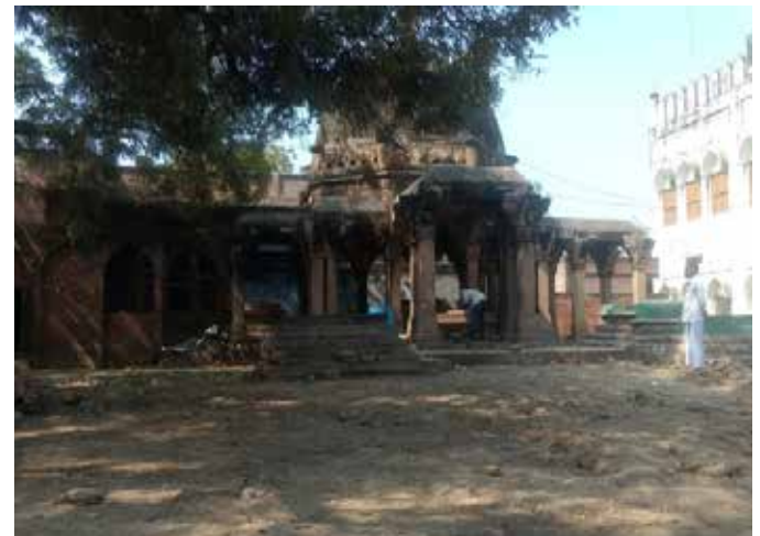
Bhattis Khamba- Before Repair
