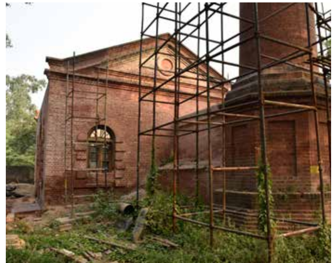
Ongoing conservation work at the colonial period pump house at 40 Khoo
