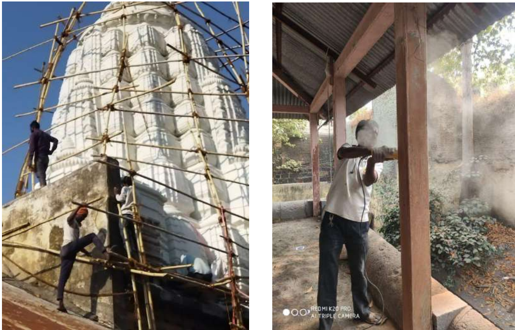
Glimpses of various conservation and restoration works being carried out on site
